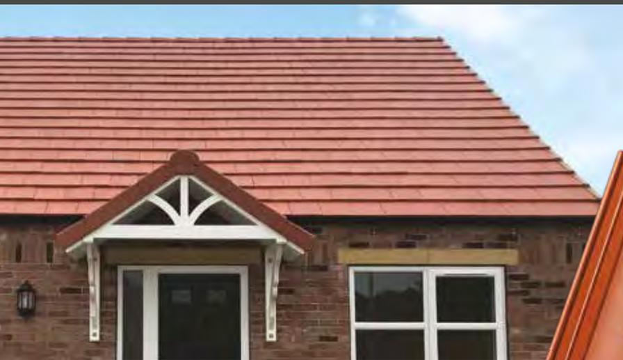
An energy conscious production process as well as a recycling concept, enhances our contribution towards a clean environment. Nelskamp concrete tiles are produced according to DIN EN 490/491 and DIN18338. The deep side-interlock provides optimal protection against wind-driven rain, snow and dust particles.
